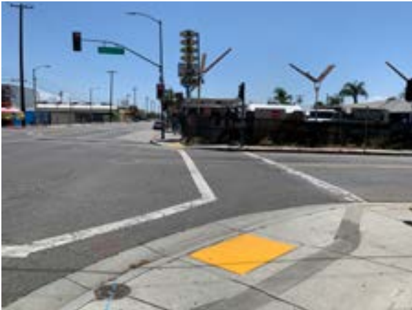
A standard crosswalk with two parallel lines and an ADA compliant curb ramp, East Los Angeles
